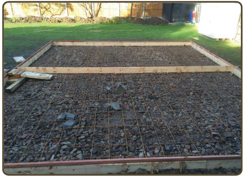
Below - Steel Reinforced concrete base for large cabins
