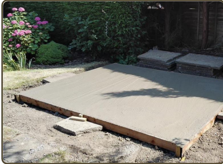
Below – simple concrete base with timber shuttering
