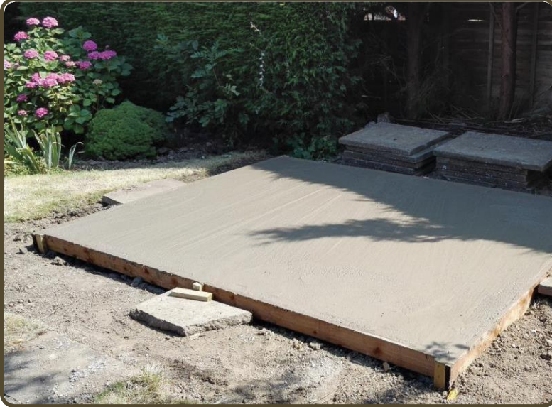
Below – simple concrete base with timber shuttering
